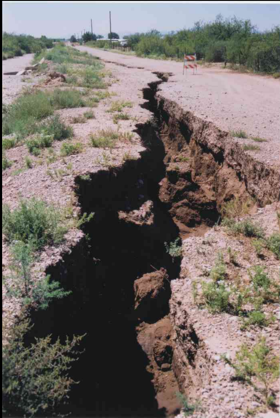
Nickels Road, looking south, 7-26-04
