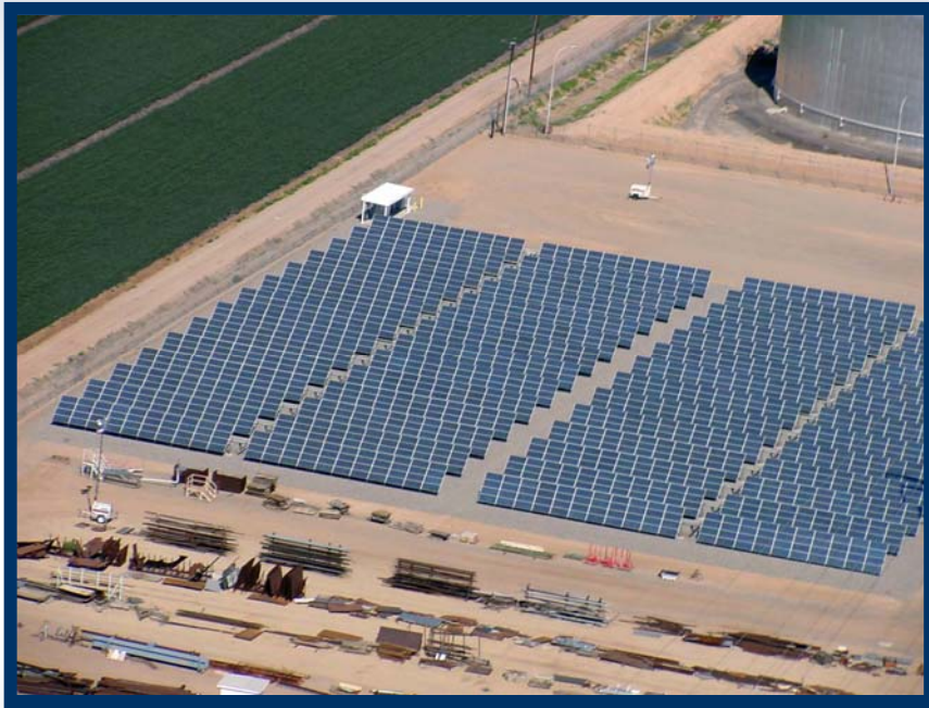
Agua Fria Generating Station, Glendale 200 kW
